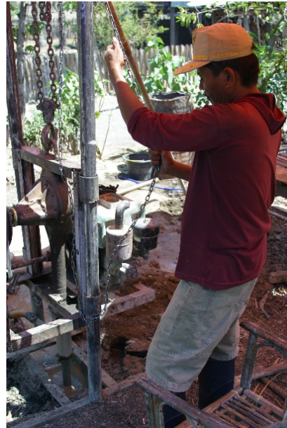
Boring for clean water
